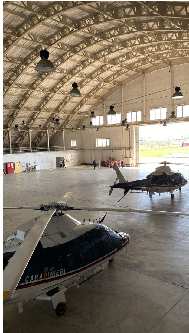
Figure 1 | Interiors of Pontecagnano Hangar.
