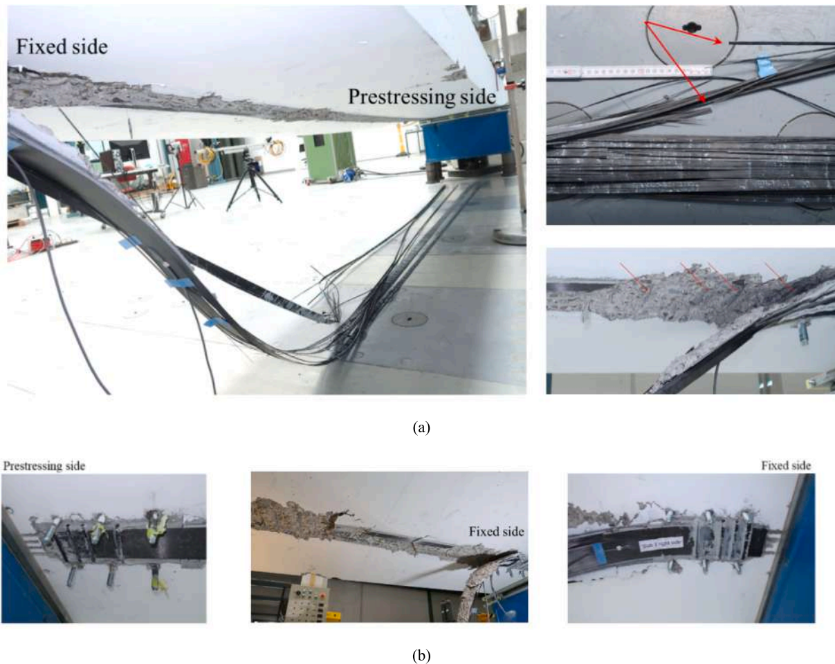
Fig. 12. Failure mode of prestressed slab (EBROG-P): (a) strip failure and cracks in the concrete below the adhesive, (b) end anchorage failure.
