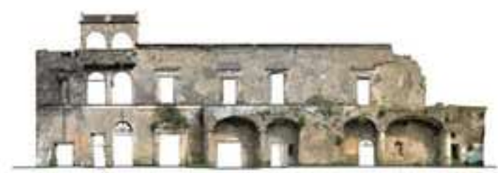
Main elevation photograph - scale 1:100
