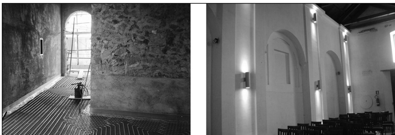
Figure 4 - “Floor” heating system (left) and LED lighting (right)
