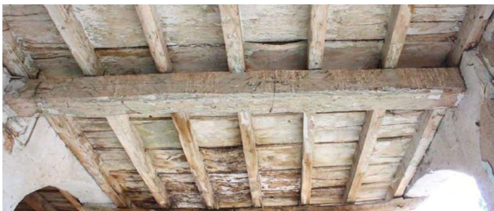
Figure 7. Internal cloister; detail of a wooden floor with a double row of beams and overlapping joists.
