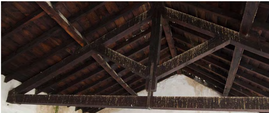
Figure 6. Gallery; detail of an open-node truss.
