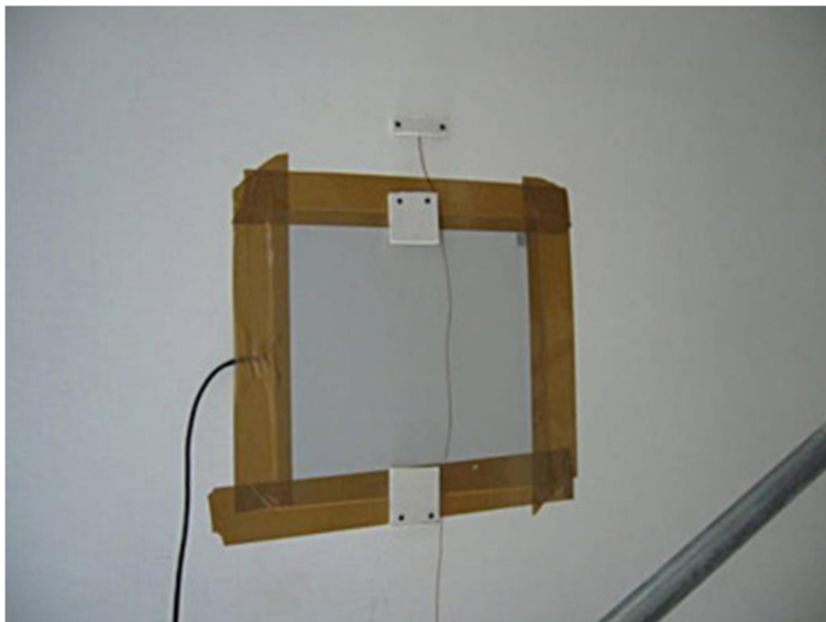
Fig. 5. The heat flux meter and one of the temperature probes installed indoor on the south wall for the measurement of thermal transmittance.
