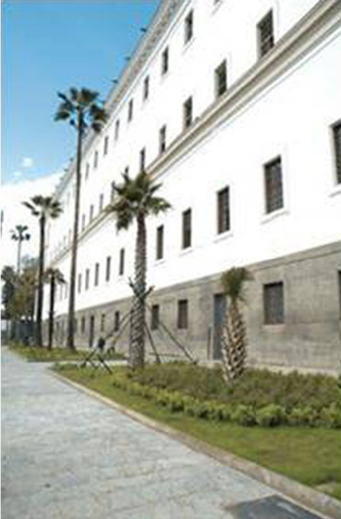
Fig. 3. The building facade.
