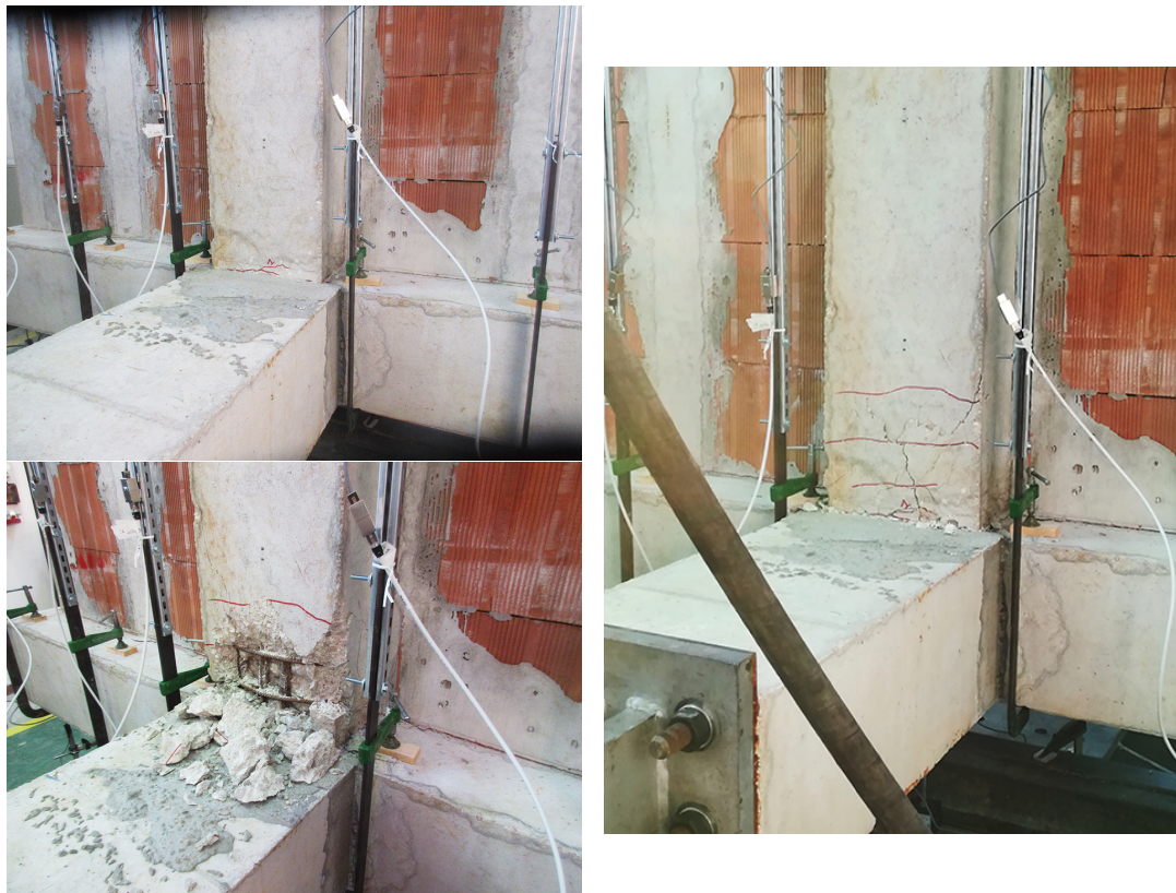
FIGURE 4.38: Crack pattern evolution on the joists side of J_01_S – Geolite – C specimen.
