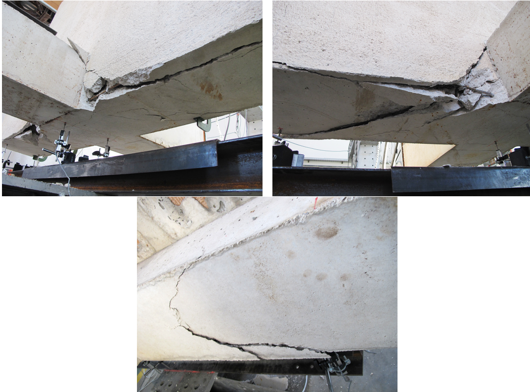
FIGURE 4.52: Crack pattern evolution in the joint and longitudinal beams of J_{01\_S} - M^- specimen.
