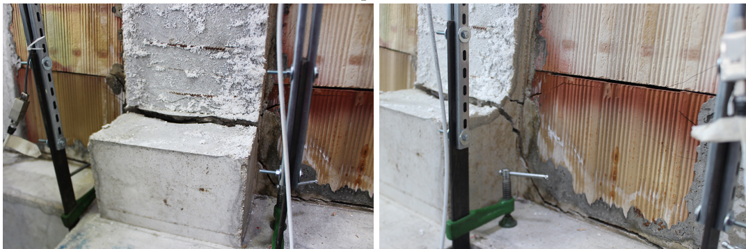
FIGURE 4.95: Crack pattern at the end of the test in the beam of J_{02\_S} - M^+ specimen.
