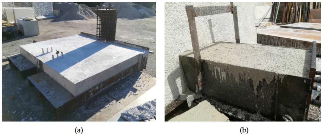
FIGURE 2.28: Concrete casting steps.
