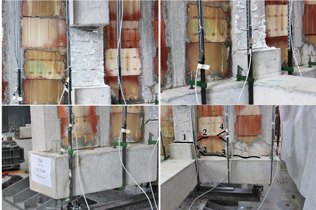
FIGURE 4.92: Crack pattern evolution on the joists side of J_{02\_S} - M^+ specimen.
