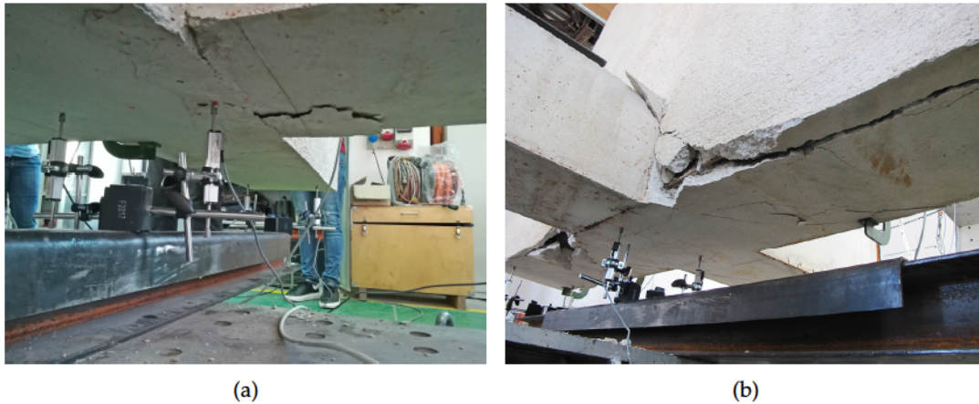
FIGURE 5.7: Longitudinal beams crack pattern in J_{01\_S} - M^+ and J_{01\_S} - M^- specimens.
