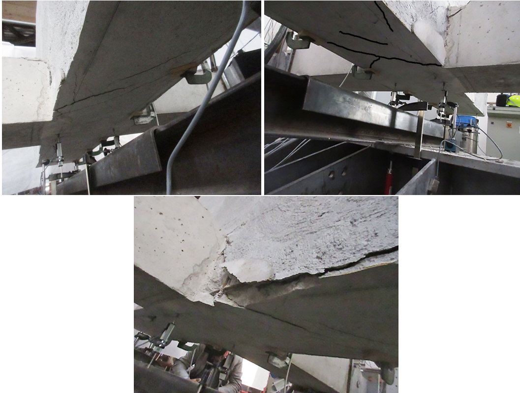
FIGURE 4.44: Crack pattern evolution in the joint and longitudinal beams of J_{01\_S} - C specimen.
