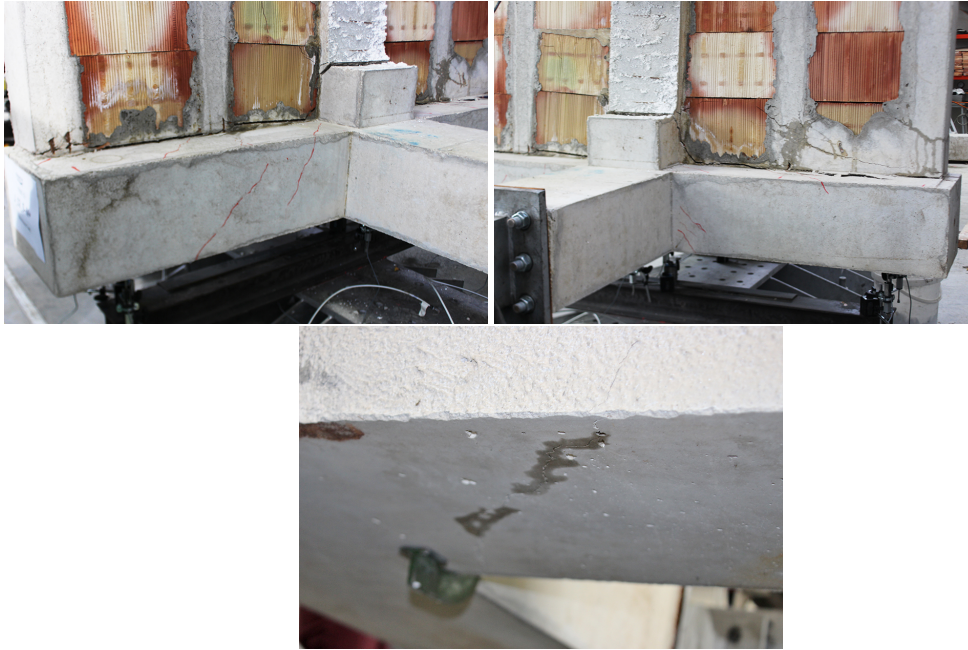
FIGURE 4.94: Crack pattern evolution in the joint and longitudinal beams of J_{02\_S} - M^+ specimen.
