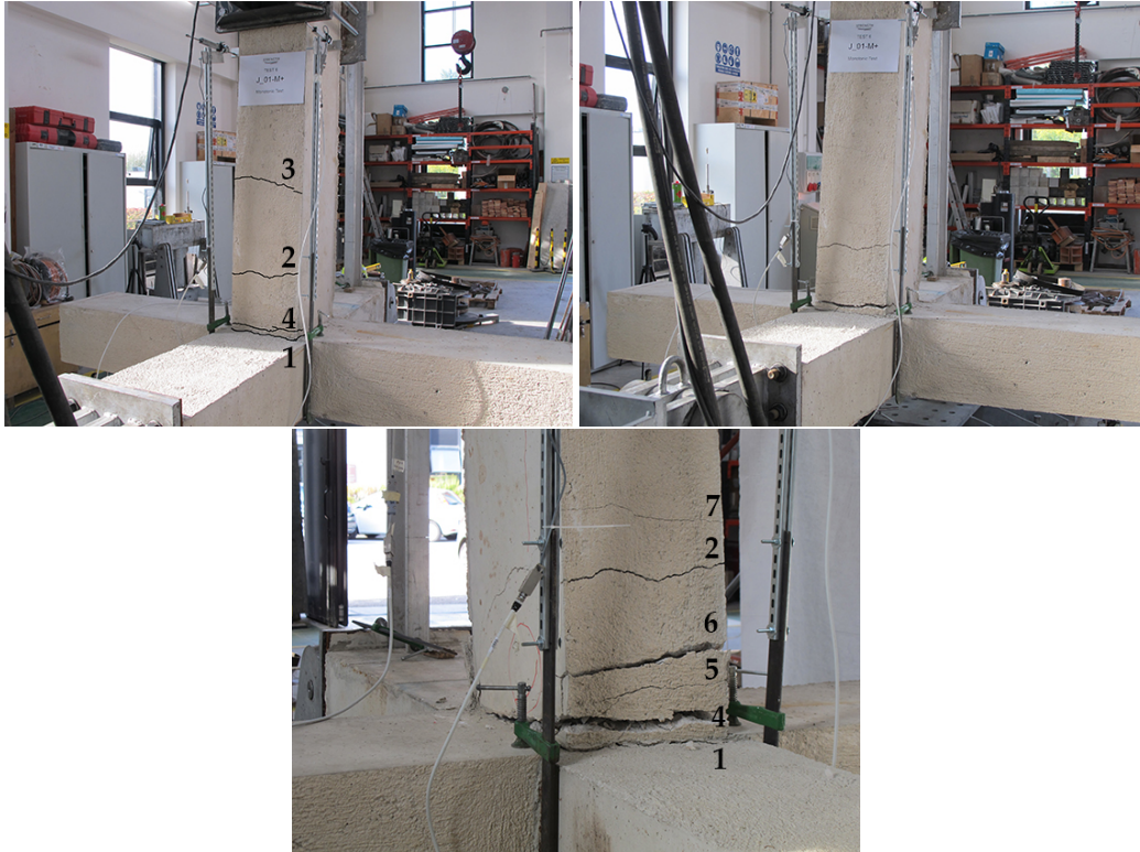
FIGURE 4.17: Crack pattern evolution in J_{01} - M^+ specimen.
