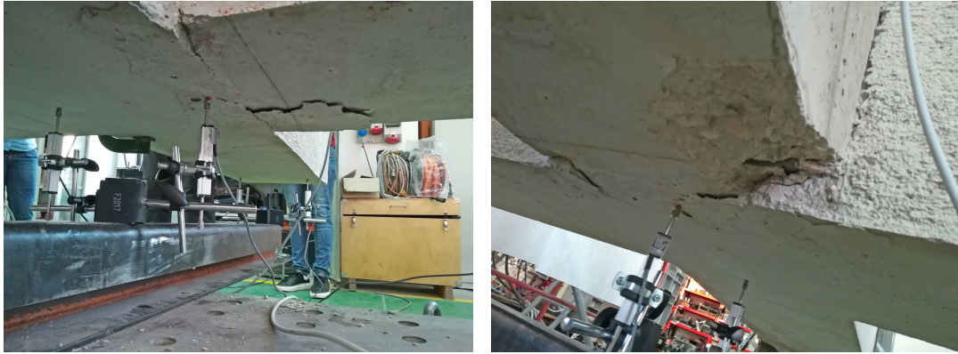
FIGURE 4.48: Crack pattern evolution in the joint and longitudinal beams of J_{01\_S} - M^+ specimen.
