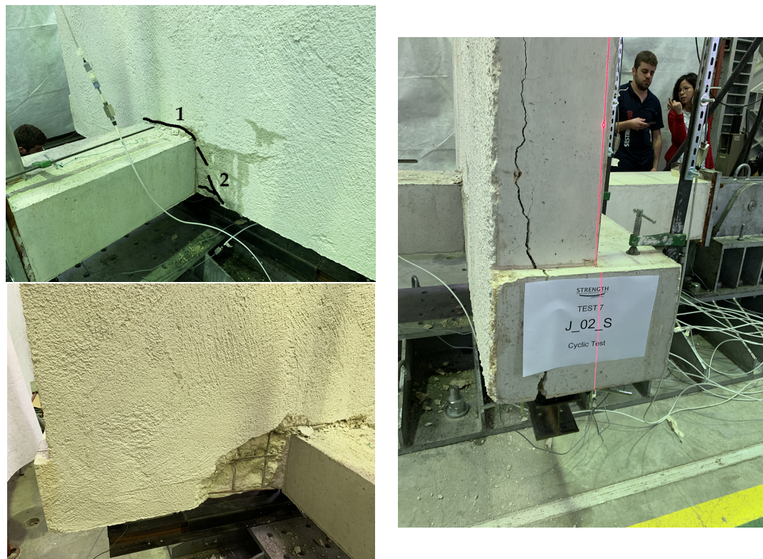
FIGURE 4.89: Crack pattern evolution on the slab side of J_{02\_S} - C specimen.
