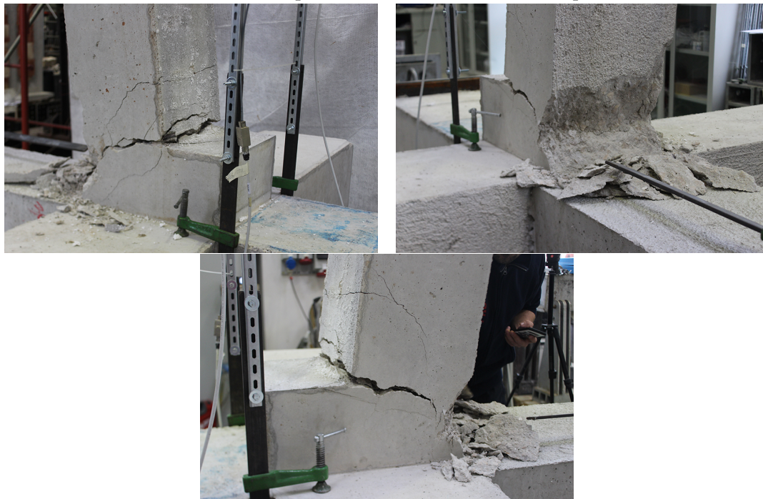
FIGURE 4.71: Final damage in the beam of J_{02} - M^+ specimen.
