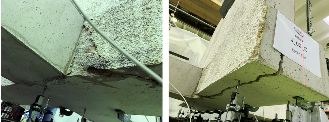
FIGURE 4.90: Crack pattern evolution in the joint and longitudinal beams of J_{02\_S} - C specimen.
