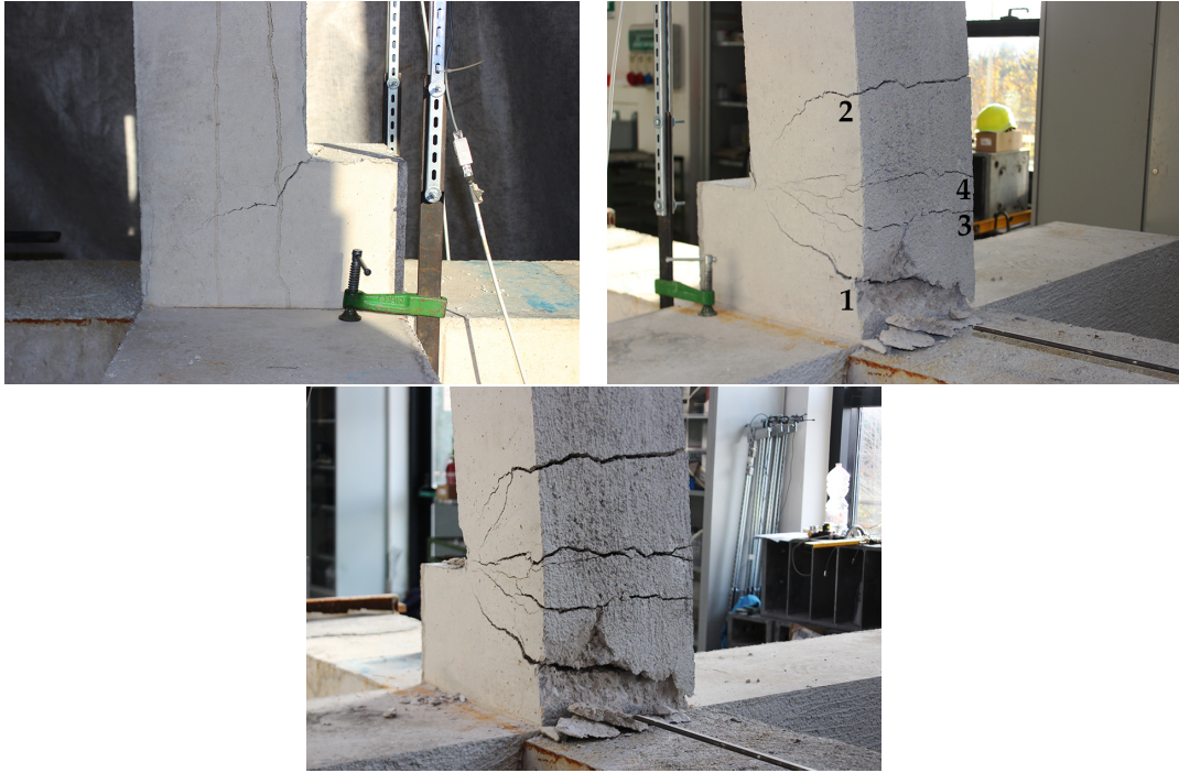
FIGURE 4.72: Crack pattern evolution in J_{02} - M^- specimen.
