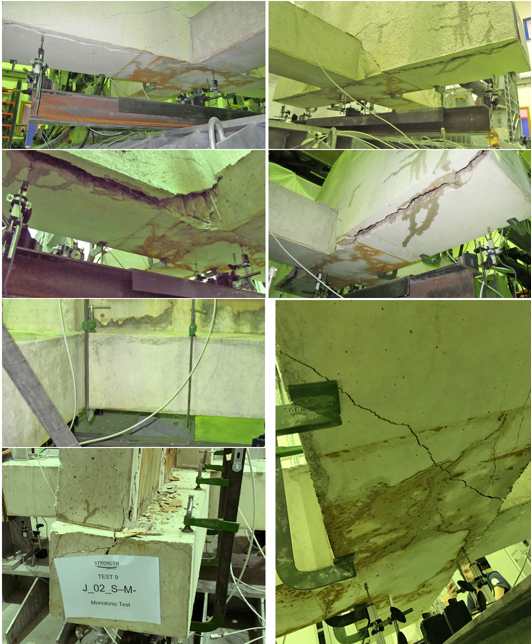
FIGURE 4.98: Crack pattern evolution in the joint and longitudinal beams of J_{02\_S} - M^- specimen.
