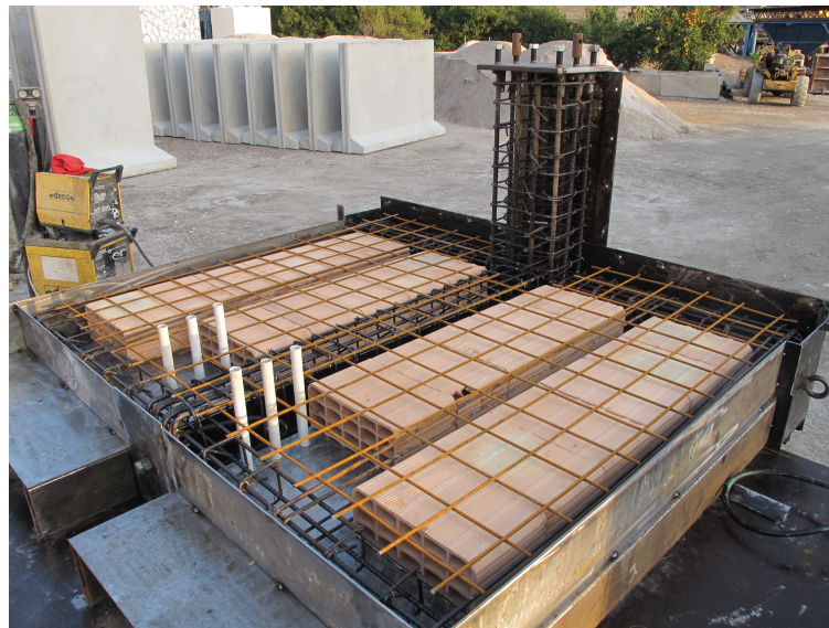
FIGURE 2.26: Reinforcement of the J_01_S module in the form-work.
